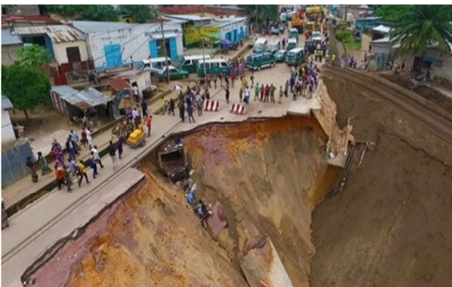
Figure 2. Erosion of Ngamakosso, destruction of traffic ways (District 6 Talangai, Brazzaville).
