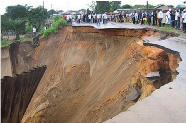
Figure 1. Erosion of Ngamakosso, roadway collapse (District 6 Talangai, Brazzaville).
